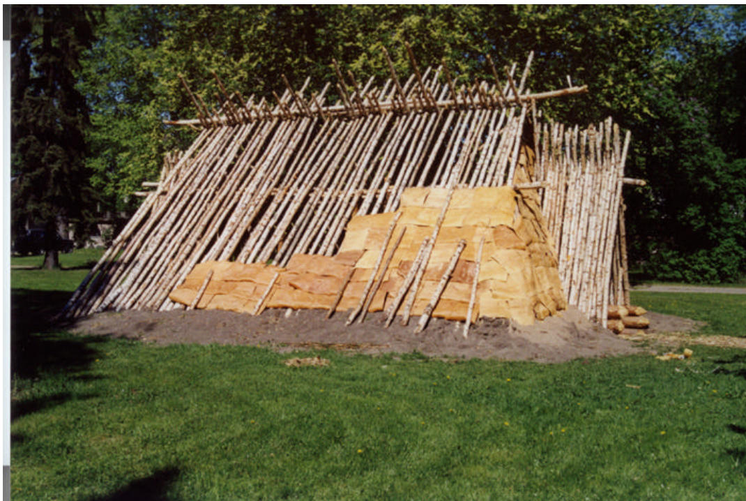
The house of Kärmelahti reconstructed in the yard of the National Museum of Finland in Helsinki (Photo Eero Muurimäki)
